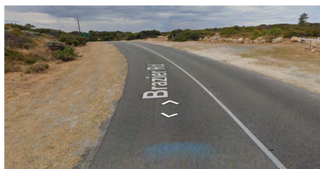
Figure 7: East-west section of Brazier Rd, looking east.
