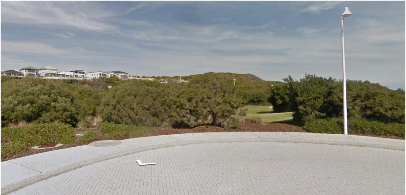
Figure 3 Streetview of subject site (Google Maps)
