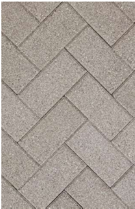
Material: Trafficable Unit Paver Colour: Natural dune / silver sand tones Location: Shared parking and pedestrian-priority areas
